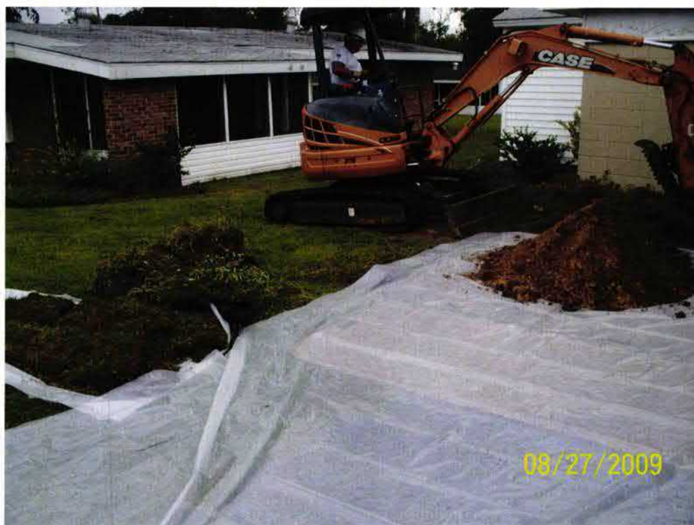
Picture 2: UST 1243Dove removal in progress.
